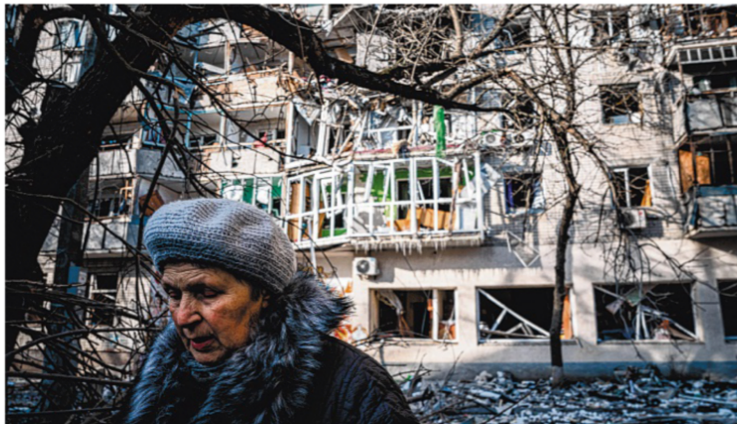
A damaged residential building in Kherson, Ukraine. The Russia-Ukraine conflict has demonstrated that the consequences of major wars are impossible to anticipate and too big to ignore. PHOTO: AFP
