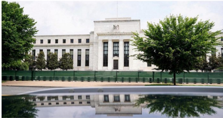
The Fed could begin lowering interest rates as soon as July, going by recent statements by Fed officials Christopher Waller and Michelle Bowman. PHOTO: REUTERS
